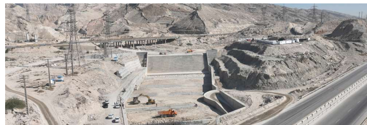
• Concrete Bed Stabilization Dam (Bedsill), Hanwies River
