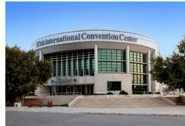
• Kish International Conference Center Building
