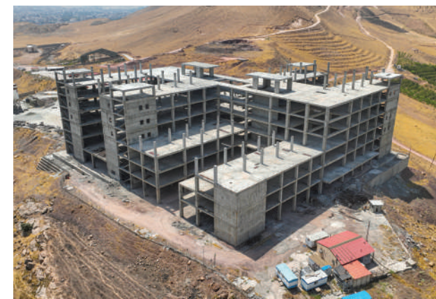
• 350-Bed Mahabad Hospital Project
