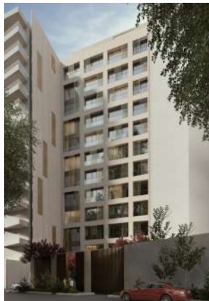
• Parsa Project, in collaboration with Sefi Construction Group
