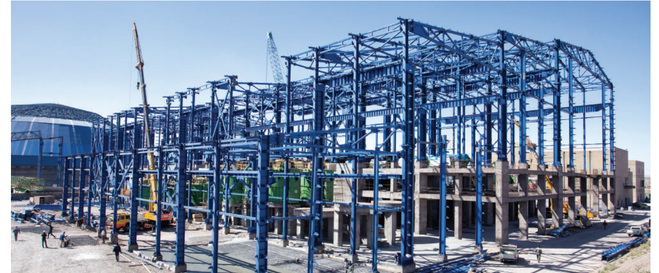
• Steel Structure for Main Hall of Sangan Iron Ore Mine Project | 4,000 tons
