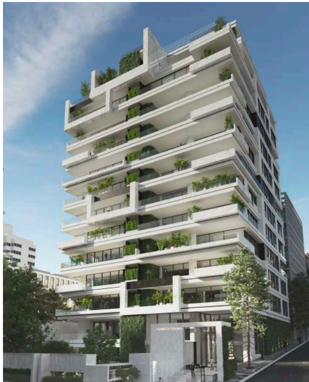
• Persian Garden Project, in collaboration with Lotus Construction Group
