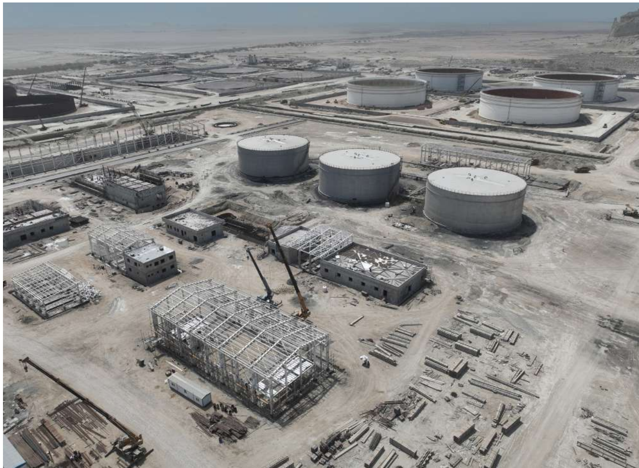
• Jask Crude Oil Storage Tanks Project
