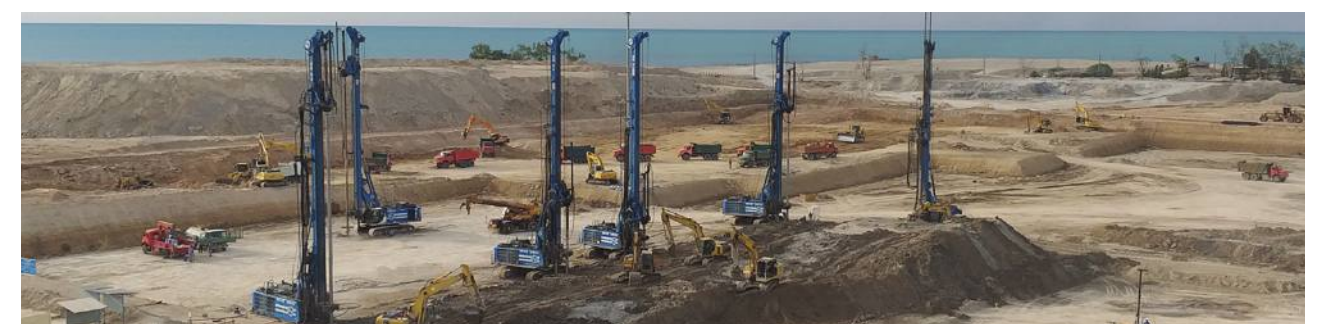
Bushehr soil stabilization project
