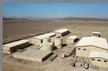
Coal-fired power station of Tabas First Coal-fired power station in Iran
