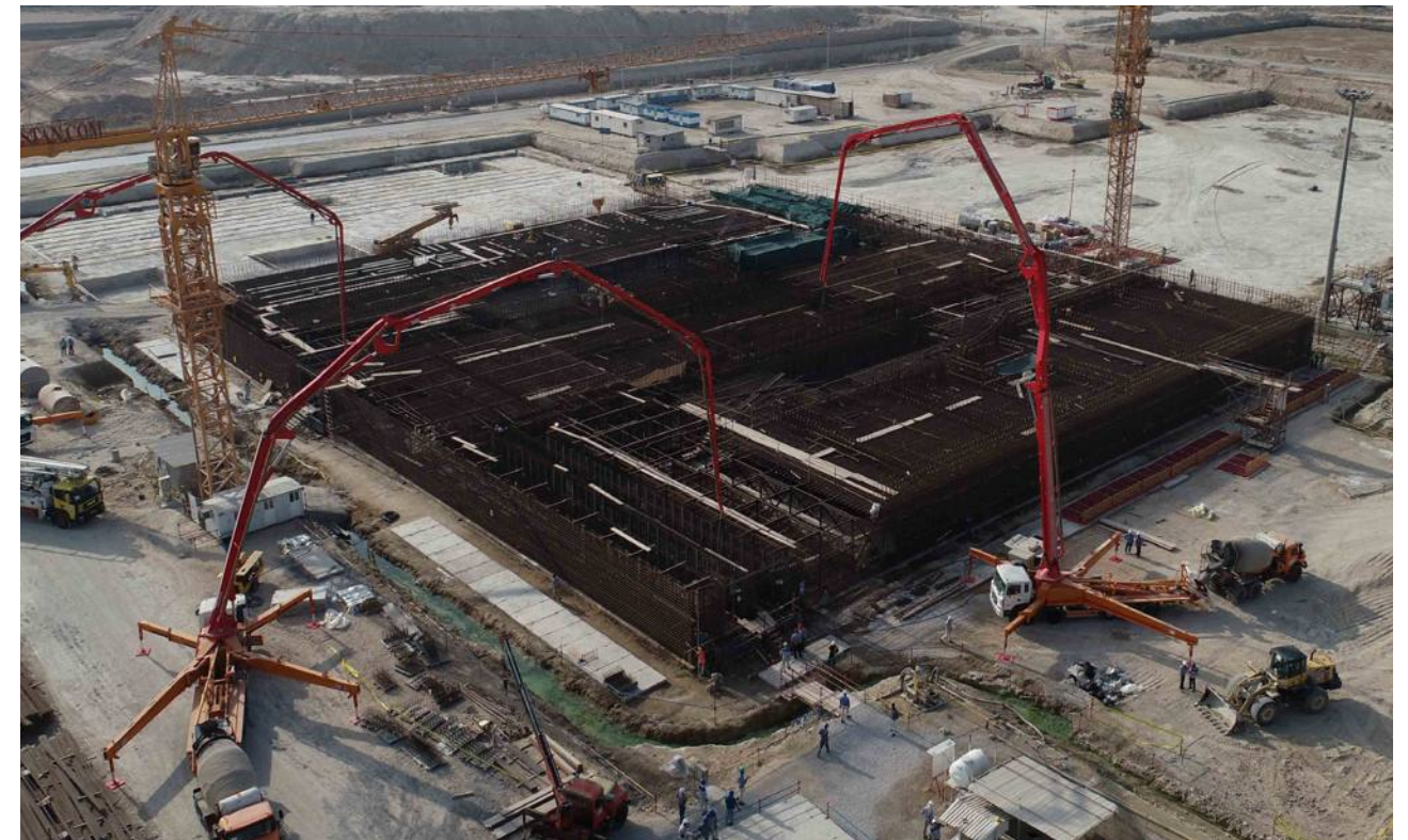
Bushehr soil stabilization project
