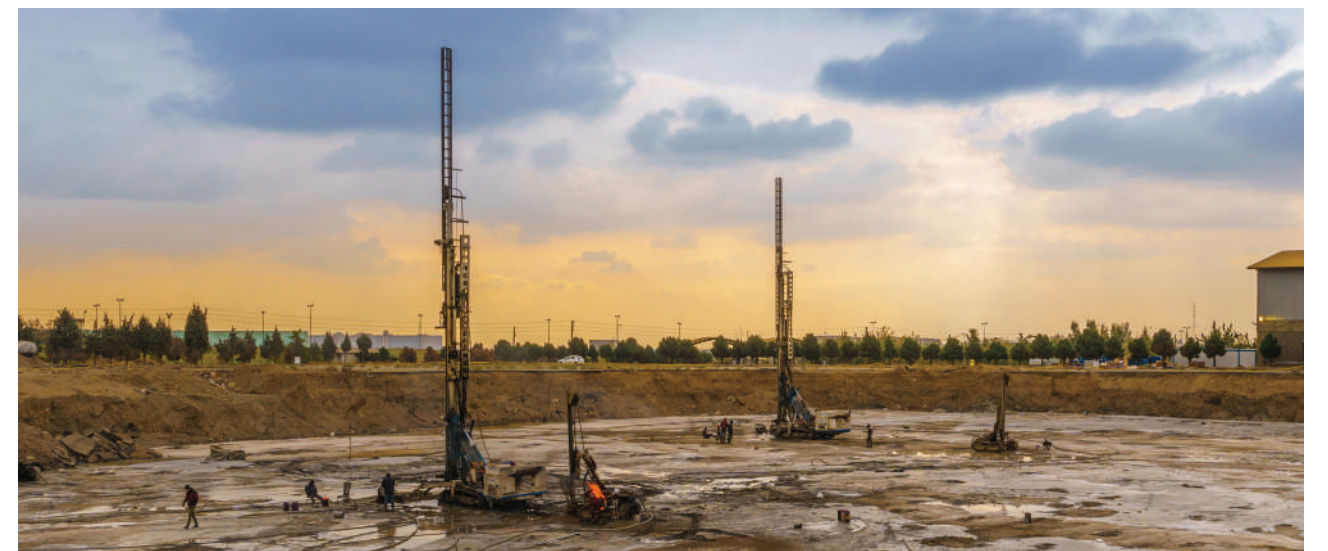
• Jet Grouting Soil Improvement for Refah Chain Store
