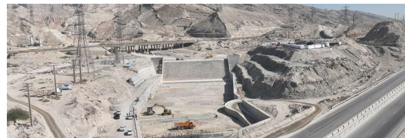
• Concrete Bed Stabilization Dam (Bedsill), Hanwies River
