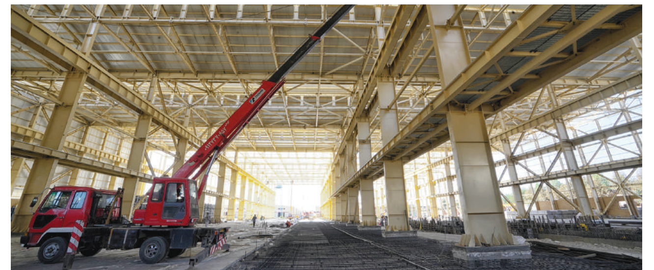
• Construction of Press Shop for Bahman Motor Company | 4,000 tons
