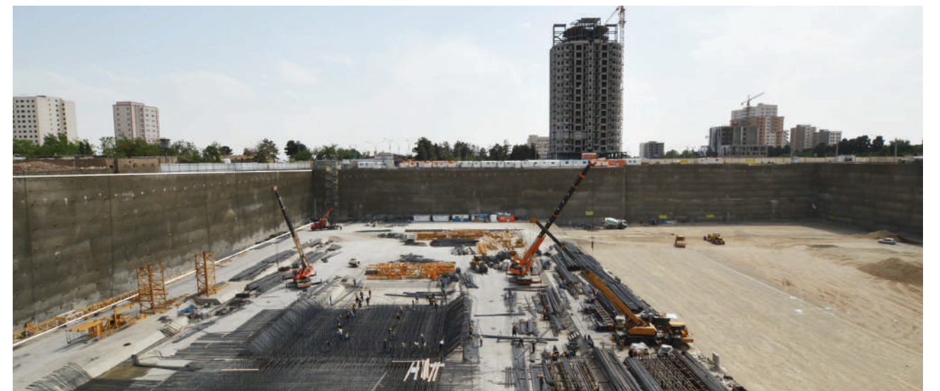
• Salamat-Barakat Hospital Project
