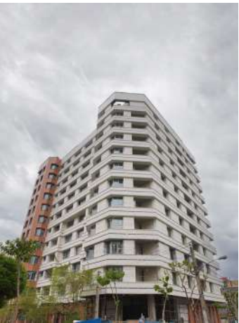
• 42-Unit Ajoudanieh Residential Complex
