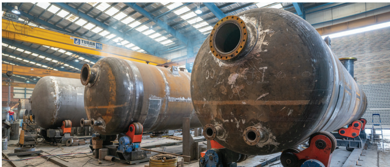
• Sand Filter Construction for Bandar Abbas Water Desalination Project | 700 tons
